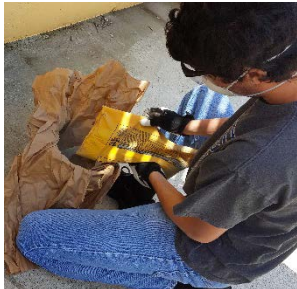
Figure 31: Donovan pouring the concrete
