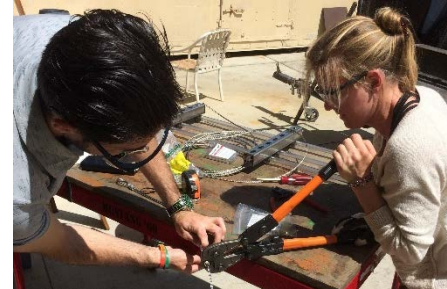
Figure 30: Christian and Dakota crimping the stainless-steel wires to the Unistruts
