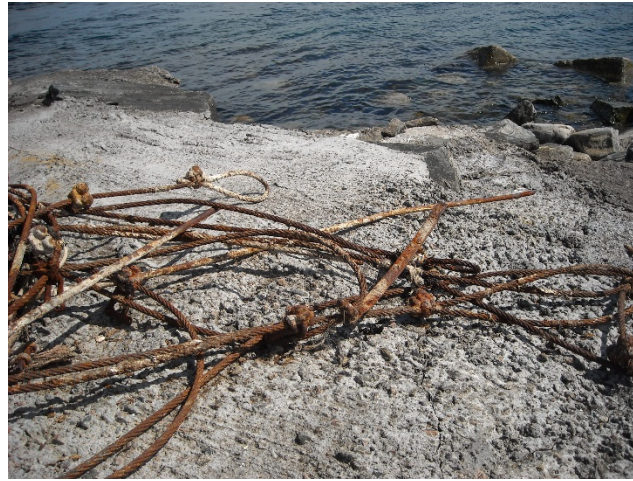
Figure 7: A 10-year old anchor cable network used for bubble curtain anchoring applications at Ringhals Nuclear Power Plant
