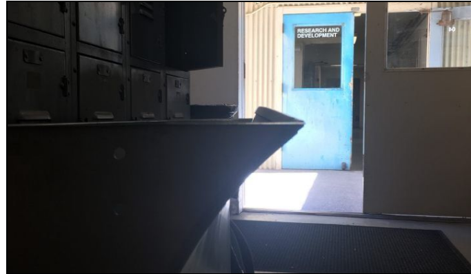
Figure 21. Side profile of plenum showing the raised back edge
