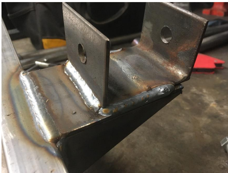
Figure 51. Supporting brackets and hinge brackets fully welded
