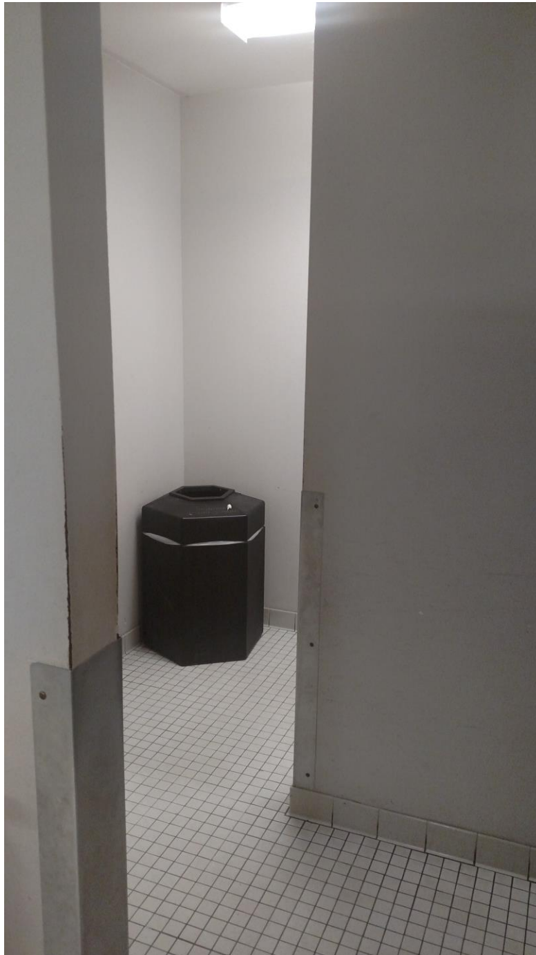
Figure 13 - Men's Locker Room Egress
