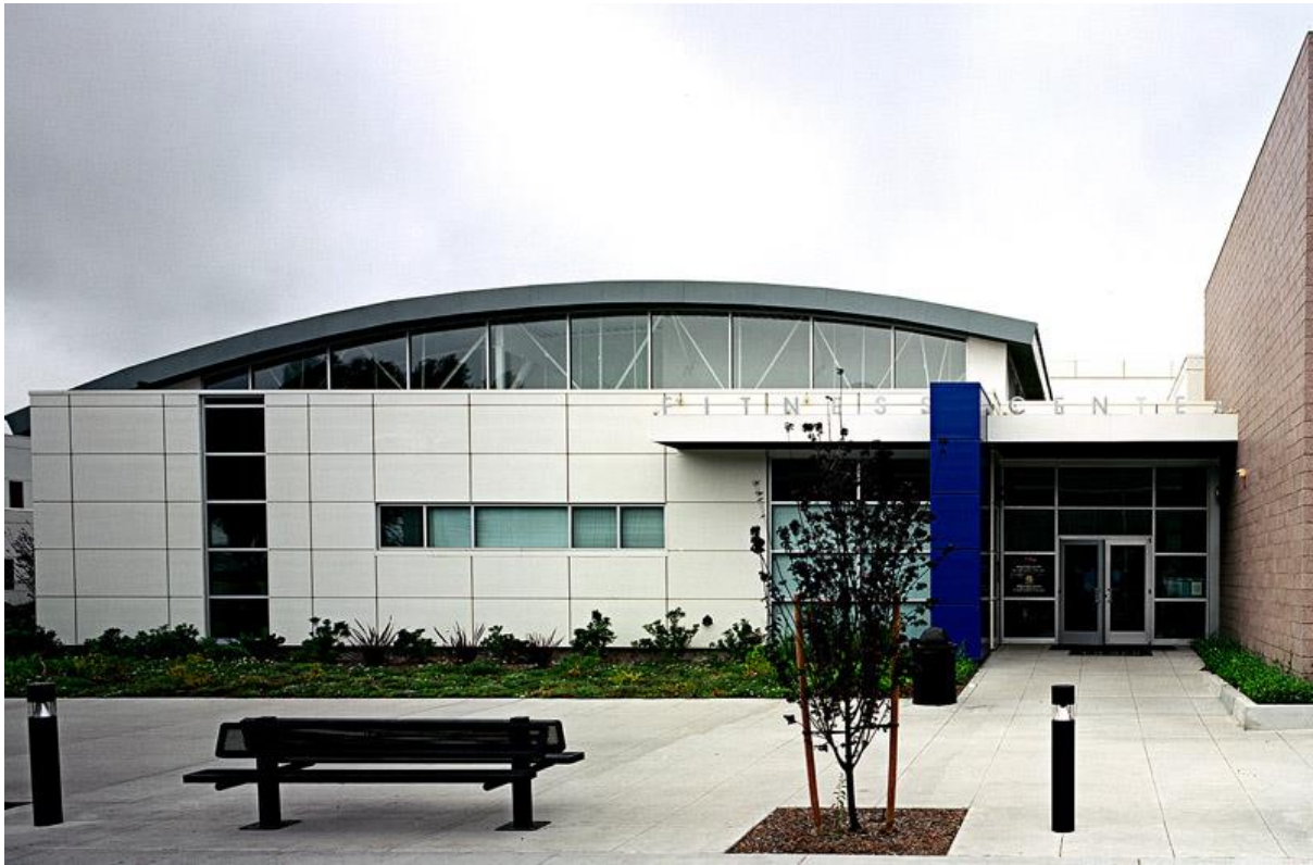
Figure 6 - Main Entrance (East Elevation) Looking West
