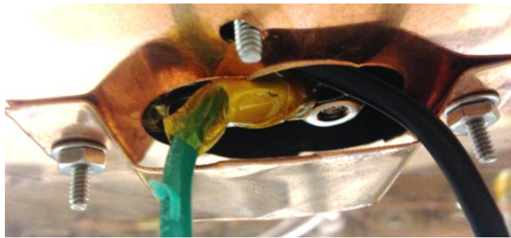
Figure 28. Copper Shroud Heater Cut Out
