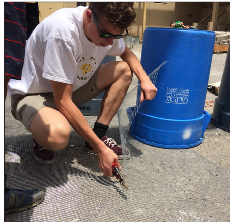
CUT AND LAY WIRE MESH
