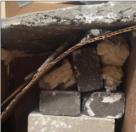
BUILD BOTTOM FORMWORK
