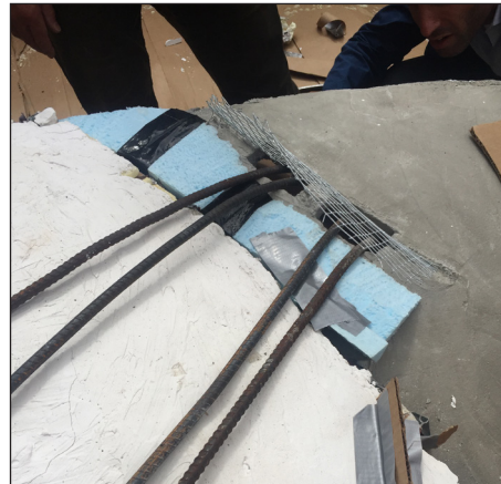
BEND AND LAY REBAR
