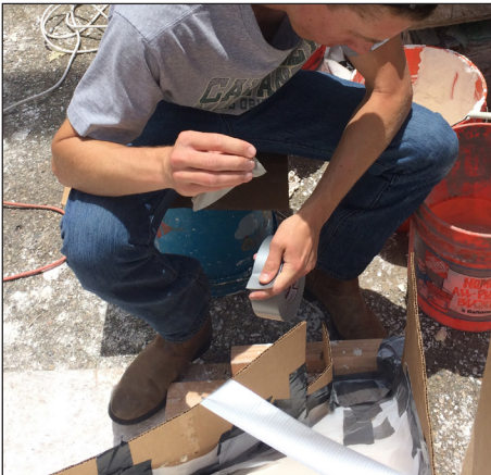
SECURE FORMWORK
