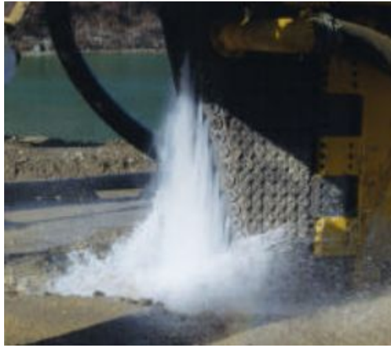
Figure 2. Jetting system stationed in front of the plow.
