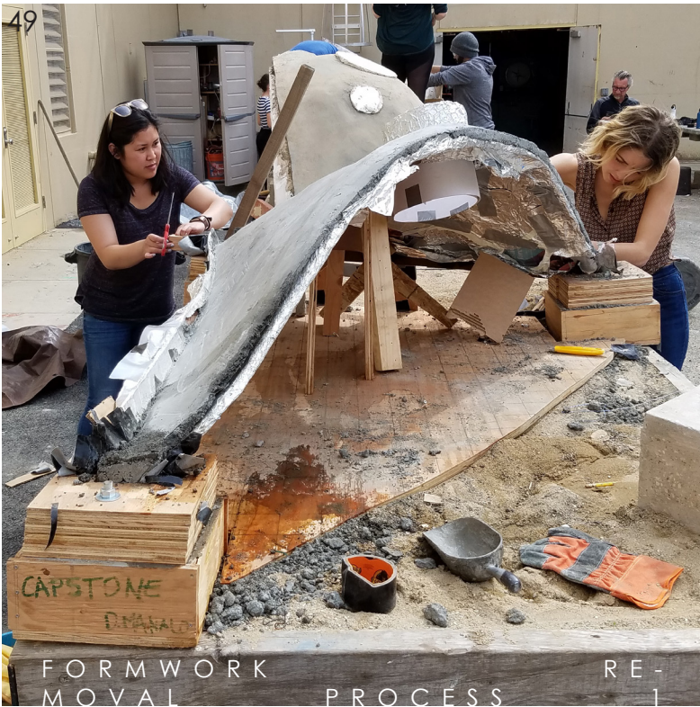
FORMWORK REMOVAL PROCESS 2
