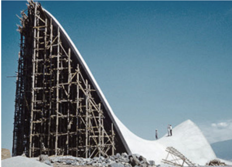
Felix Candela's Timber Formwork
