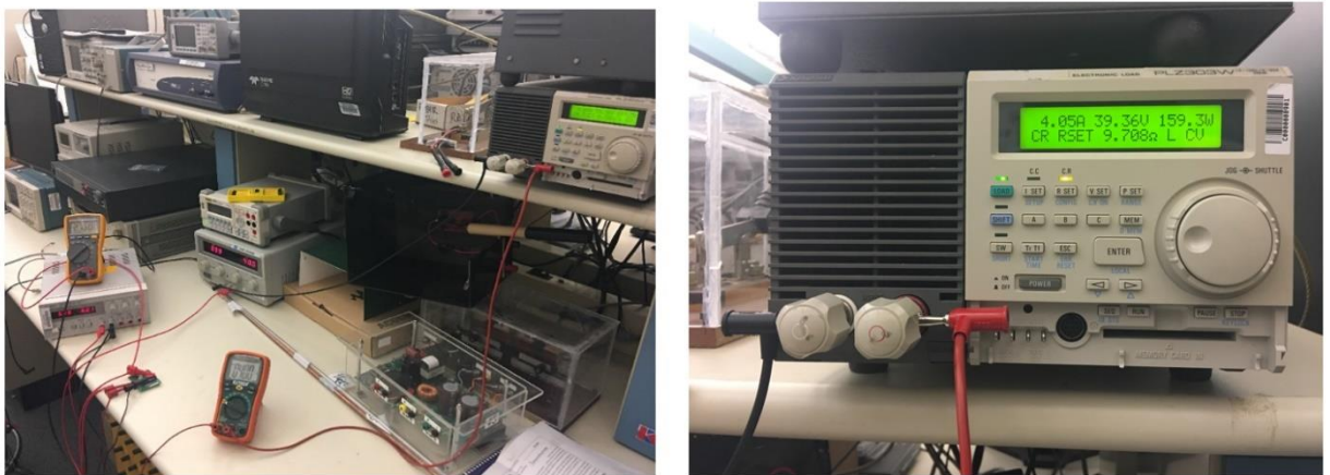
Figure 4-22 Current Sensor Testing
