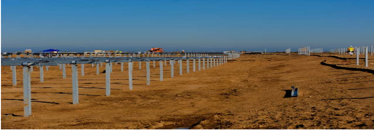
Figure 5: Dillard Solar Farm Under Construction in 2011
