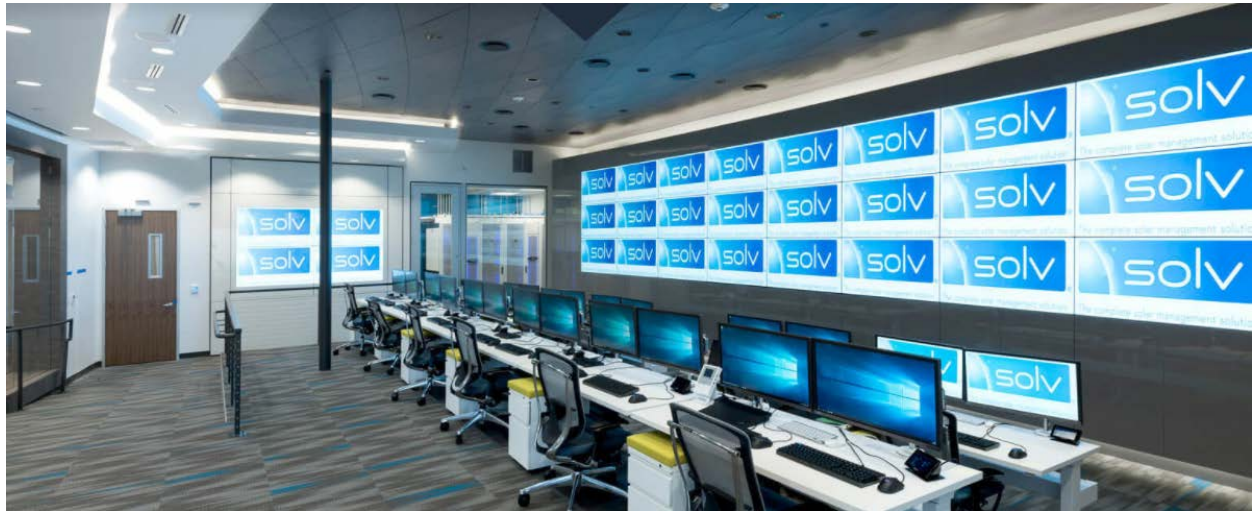
Figure 4: The Nock, SOLVs' Main O&M Center
