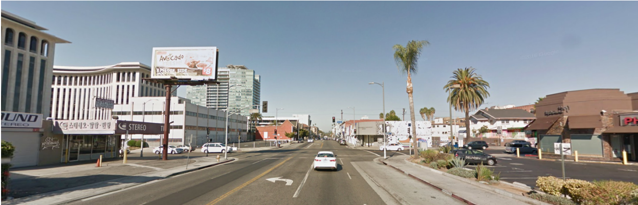
Figure 2: West 6 th Street & South Serrano Avenue
