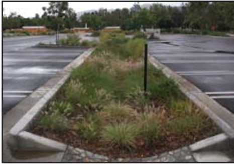
Bio-swale and curb cut example.
