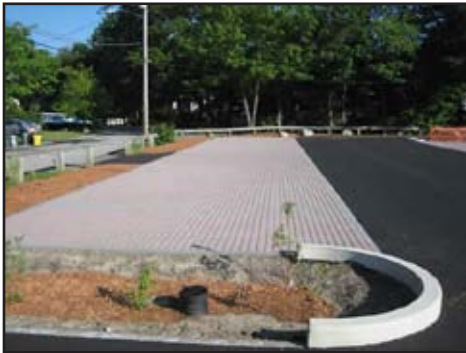
Permeable paver parking area.
