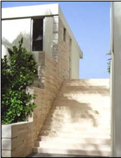
Illustrative photo of enclosed stairway.
