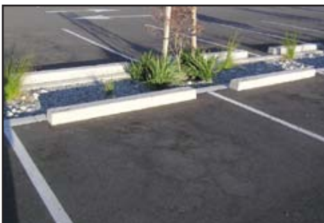
Wheel stop and bio-swale example.
