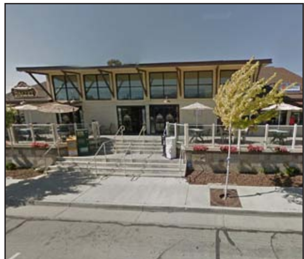
Example of terraced business front.
