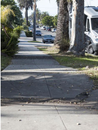
Bad example of sidewalks for pedestrian circulation
