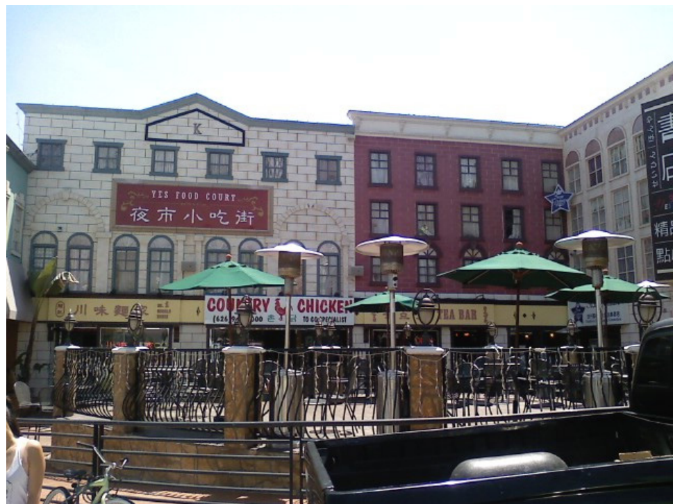
Figure 3.10 Example of great building design and style, but poor promotion leading to a “dead” corner
