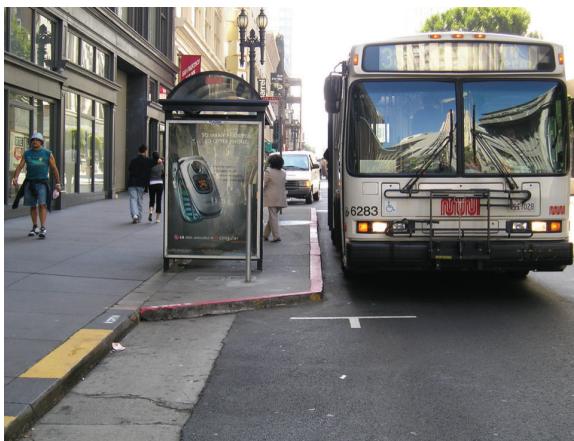
Example of bus stop loading zone that is undistruptive of normal traffic flow
