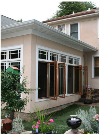
Replacement windows should be consistent with the building's architectural style
