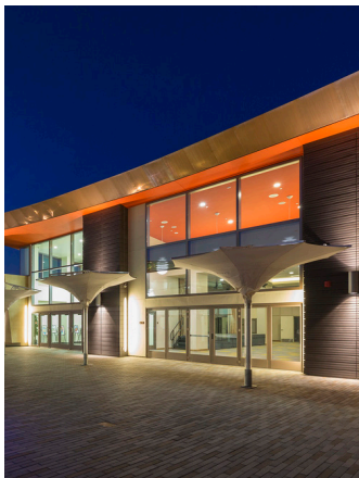
Example of good integrated building lights that eliminate glare or light spillage
