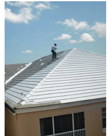
Reflective roofs are discouraged
