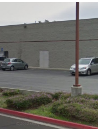
Commercial/retail loading zones shall be placed in way that minimizes visual conflict
