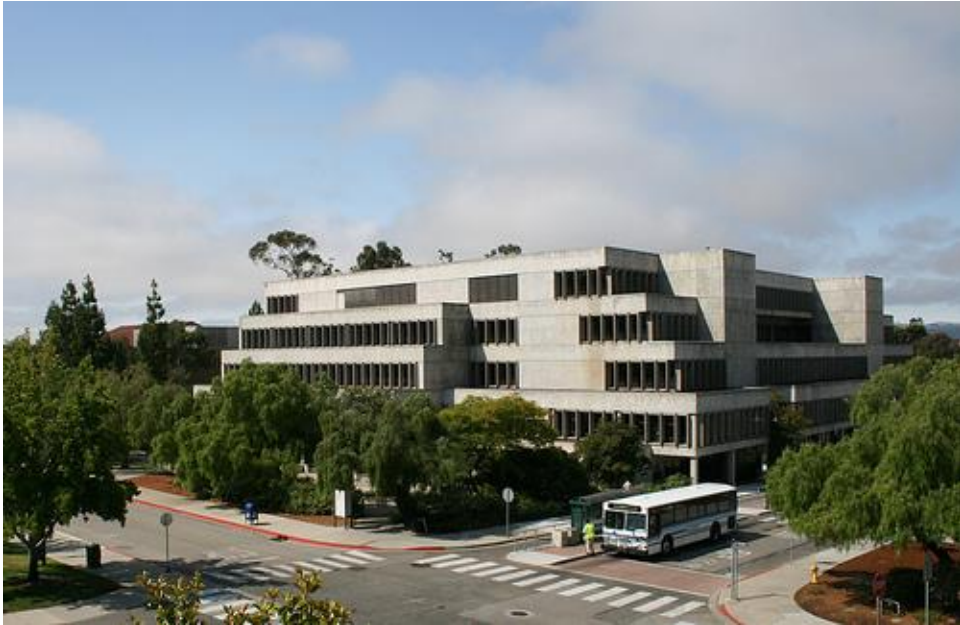
Figure 2 Back side of the Library
