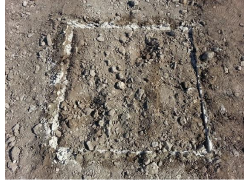
b) Remaining Bentonite Seal after the Collar Removal
