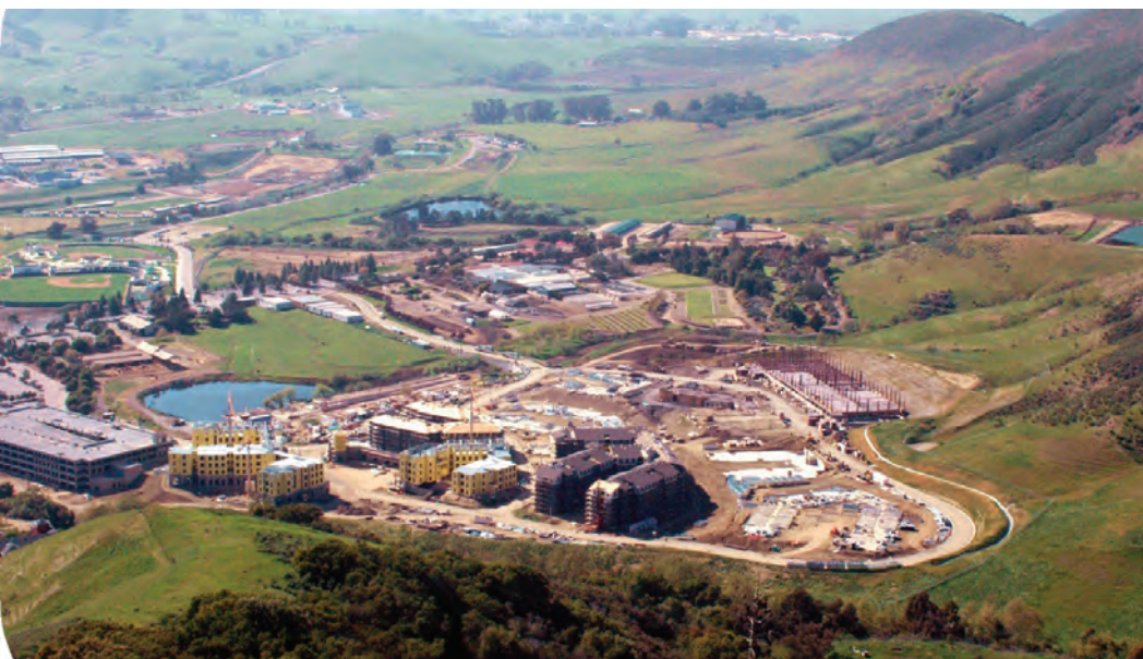
Figure 1: Poly Canyon Village. The newest student residences in the construction phase. (photo: Kevin Waldron)
