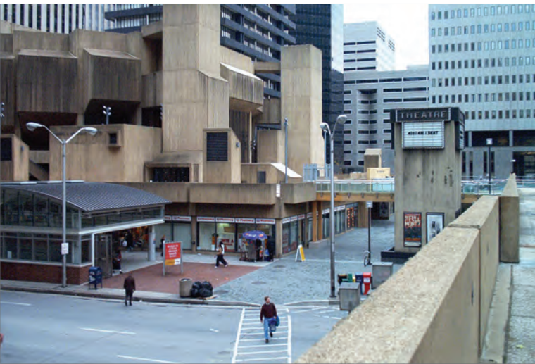
Figure 6: Getting to the south superblock from the "skywalk": the Morris Mechanic Theatre on the left, Hopkins Plaza, and the Federal Building in the background. (photo by the author, 1986)
