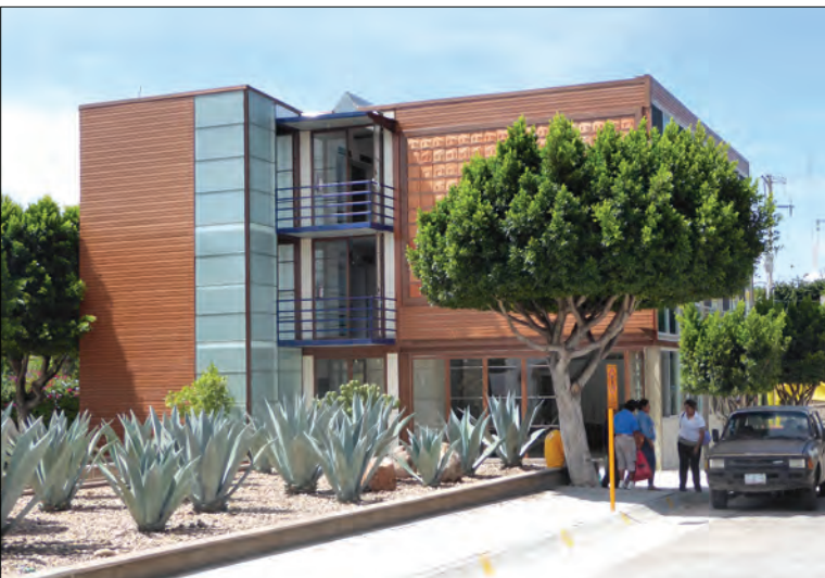
Figure 4: Los Arcos includes comfortable accommodations for students built from repurposed containers.
