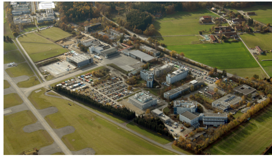
Figure 1.1: Aerial View of the DLR site in Oberpfaffenhofen (courtesy of DLR)
