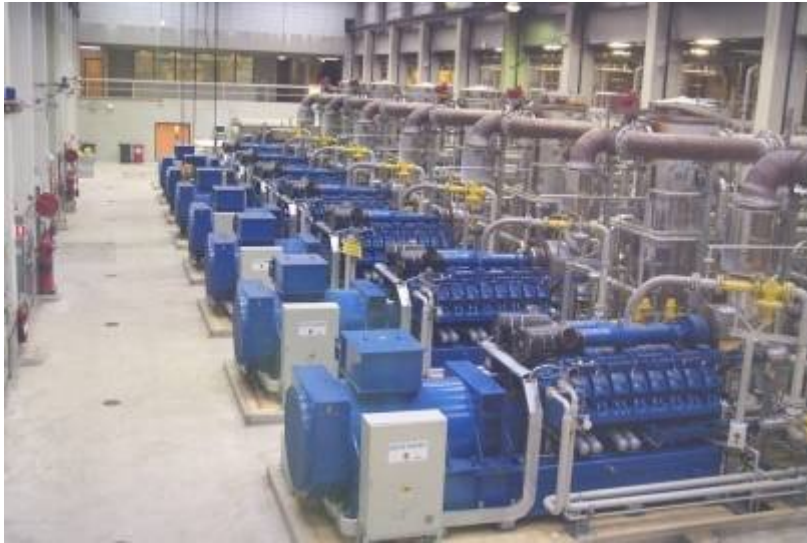
Figure 14-1 Carrum Downs biogas engine-generator sets
