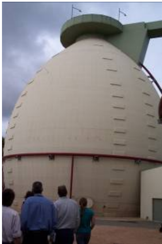
Figure 13-23 One of two egg shaped anaerobic digesters at Woodman Point, WA
