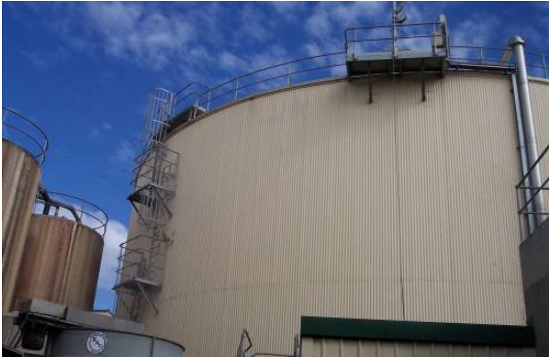
Figure 13-22 Earthpower Technologies - Sydney food digester
