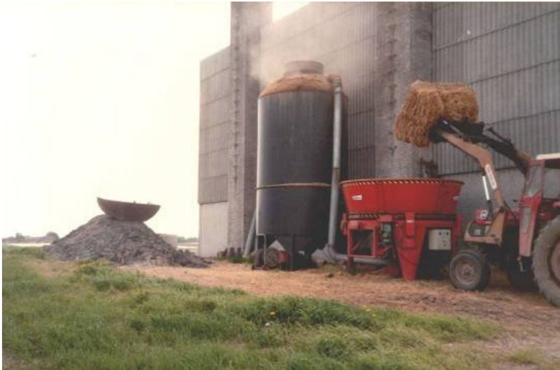
Figure 7-6 Straw bale being dropped into shredder to feed combustion plant
