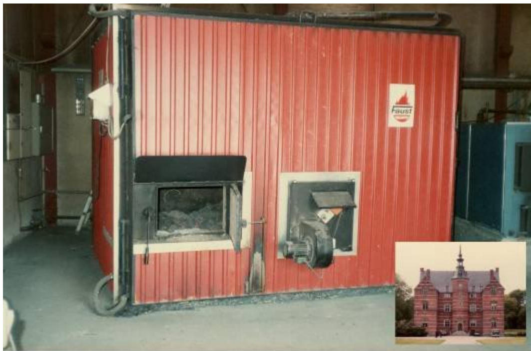
An example of one of many models of straw-fired burners as installed in Danish farms for heating the dwelling and animal houses. Note the door for ash removal.
