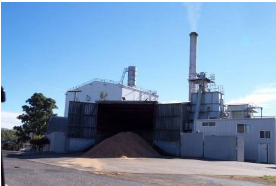
Figure 13-6 Grate boiler facility at Bega, NSW
