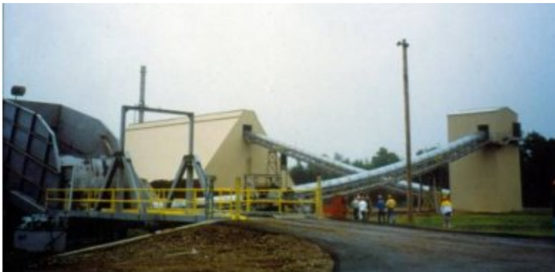
Figure 6-18 Drying a two-day supply of fuelwood occurs in the ‘A Frame’ building using waste flue gas heat at a 30MW wood-fired power generation plant in the USA
