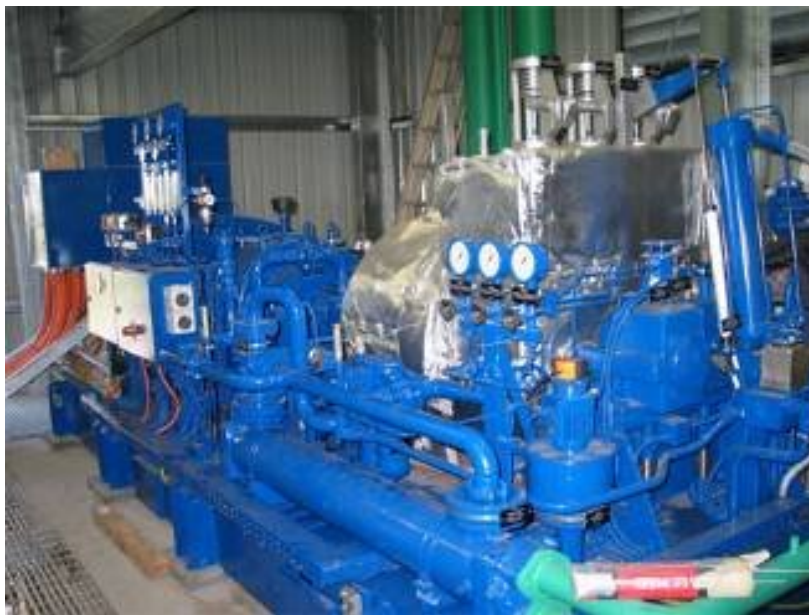
Figure 14-4 1.5 MW Steam turbine at Sun Coast Gold Macadamia, Gympie
