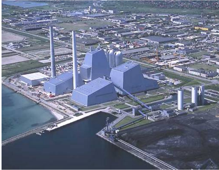
Figure 8-5 Avedore 2 combined heat and power plant
