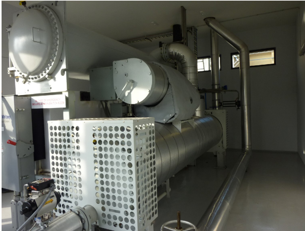
Figure 14-5 280 kW e ORC module driven by bioenergy, Gympie Timber Company
