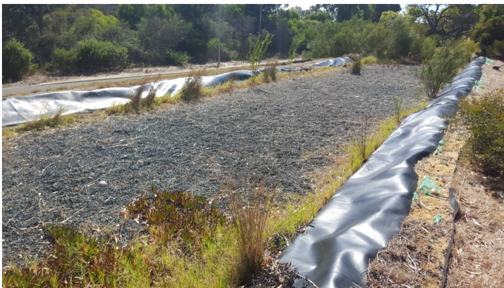
Figure 4. Image of one of the four biofilters at Timbers Edge, lacking in vegetation. Picture taken on the 26/04/16.
