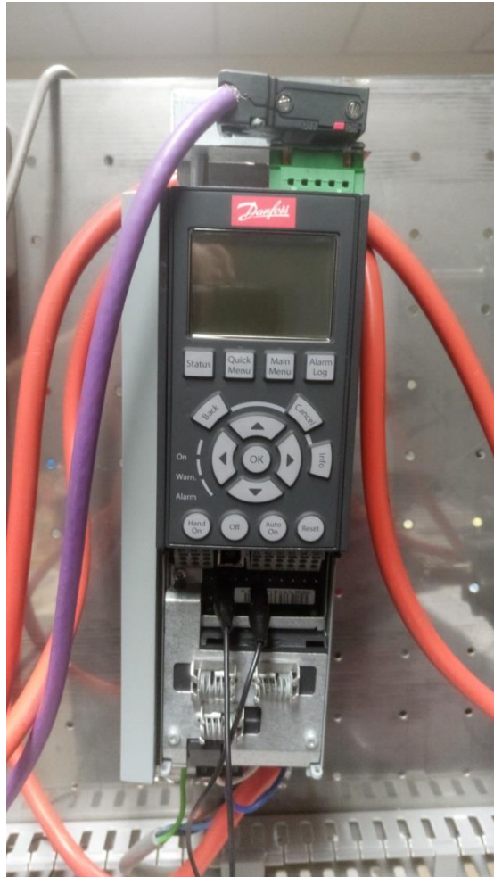
Figure 41 Danfoss HVAC FC102 VSD
