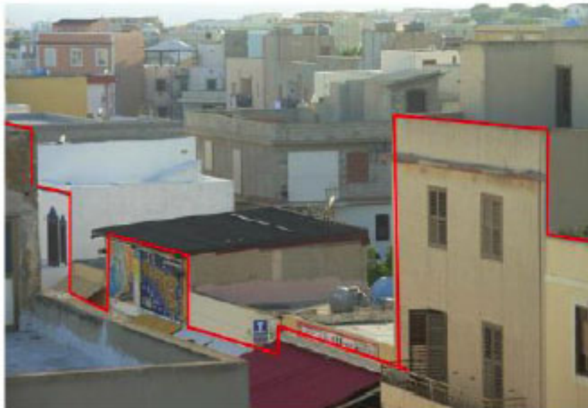
Fig. (5). Irregularity in elevation of building aggregates.
