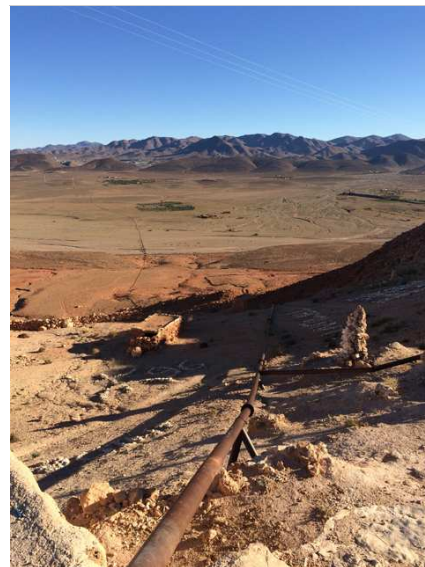
[Figure 2: The pipeline that used to provide SMI with water. Image by author.]
