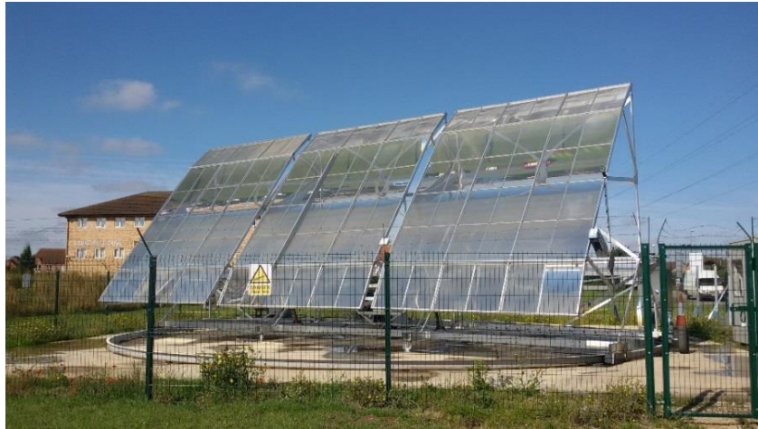
Figure 2: Experimental prototype scheme installed in Bourne, UK.
