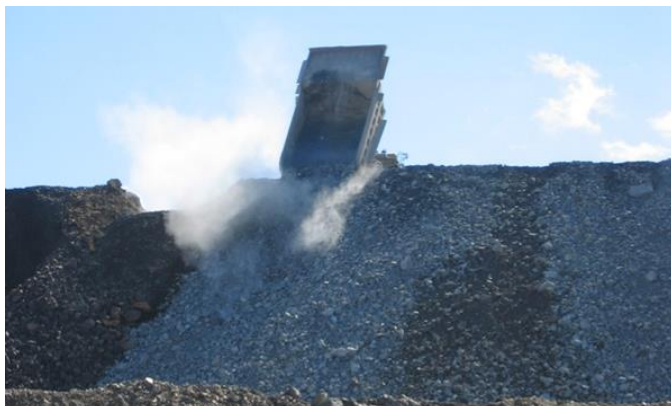
Fig. 1. End-dumping mine waste rock from a truck.
