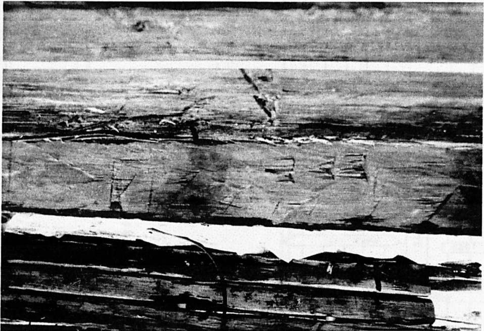
Figure 52: Photograph of tool marks on inboard side of Trent River Barge (photo: Mark Newell).
