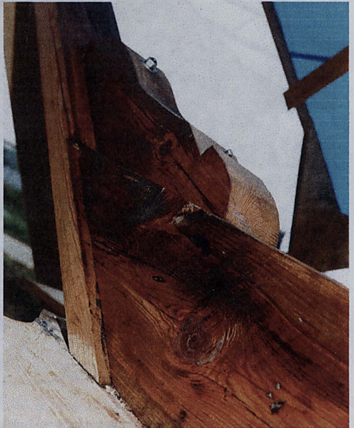
Figure 84: Above foregripe and stem knee assembly are unclamped by author after being bolted to stempost (photo: Danielle Seward) Insert - detail of assembly (photo: Mark Newell).
