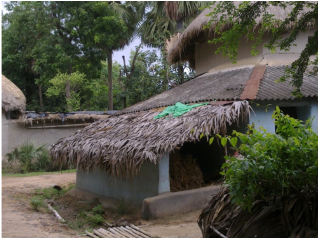
Figure 2.2: Typical house found in Kaligung and Pearson-Palli, made from bamboo or wood and mud.
