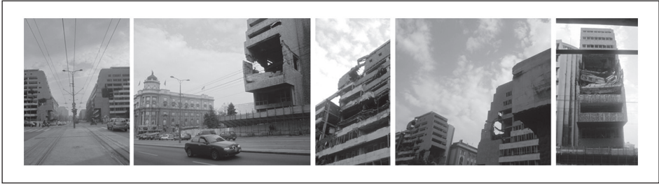
Figure 2. The Generalstab complex in (w)hole after 1999.
