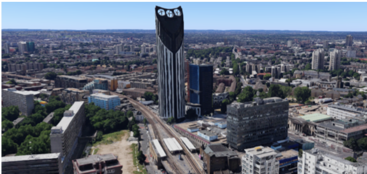
'Diving in' to understand how the developments fit in to the context of the local area
