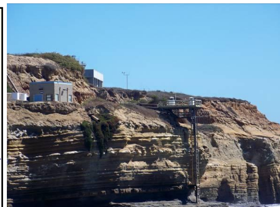
Fig. 6-3. Site seen from the shore
