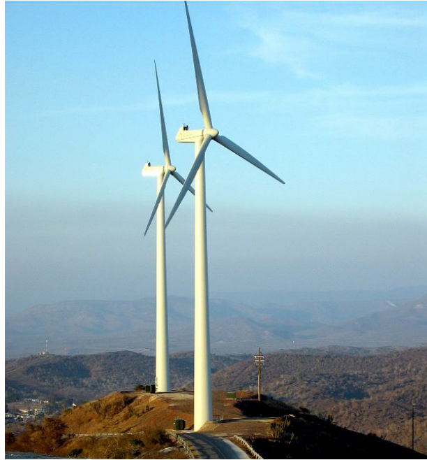
Figure 1. Wind Turbines Servicing Guantanamo Bay Naval Station. Source: [3].
