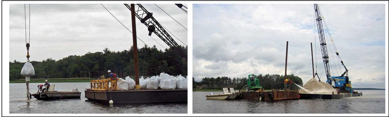
Fig. 2. Two methods used to construct reef bases. Left: mollusk shell deployed from bags. Right: shell pushed off barge at restoration site with firehose.
