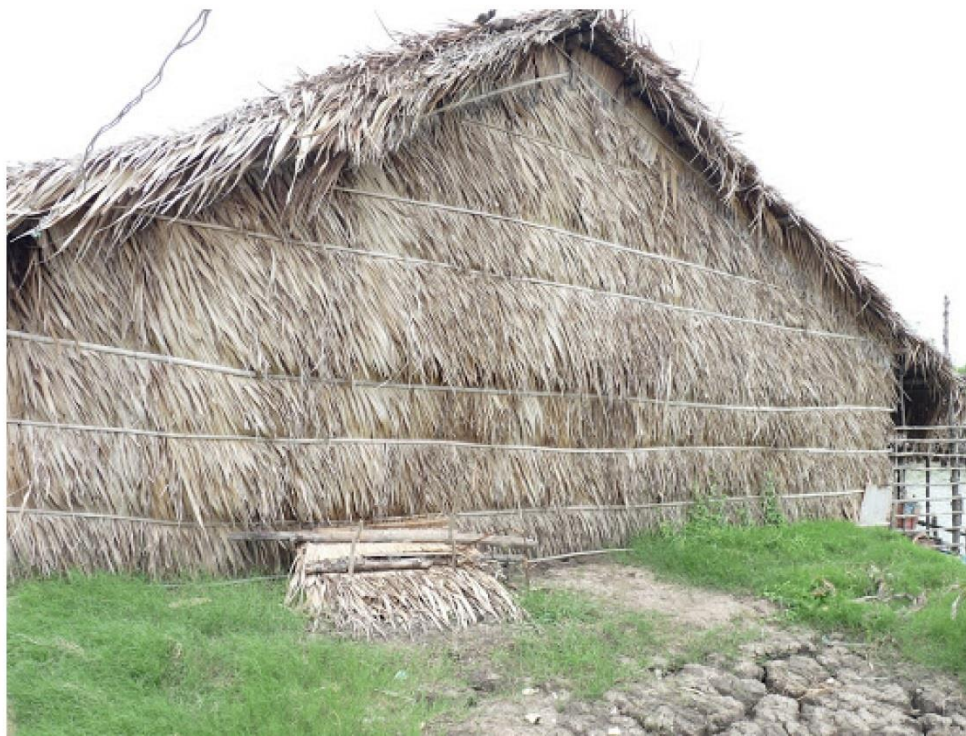
Figure 6.6 An example of coconut leaf construction as described by interviewee #2.
