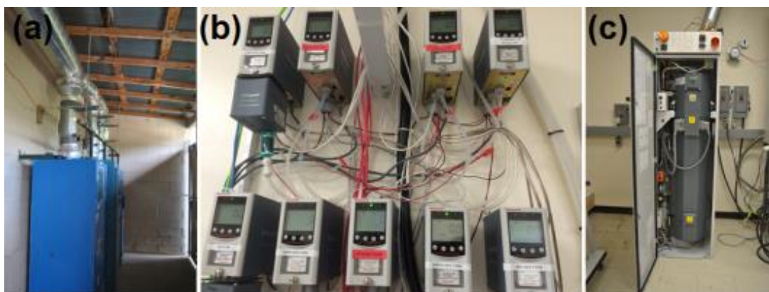
Figure 14. Safety features implemented inside and outside the lab. (a) Exhausted gas cabinet in the gas farm, (b) gas sniffers that detect inside the lab (top) and in the gas farm (bottom), and (c) gas reactor column.
