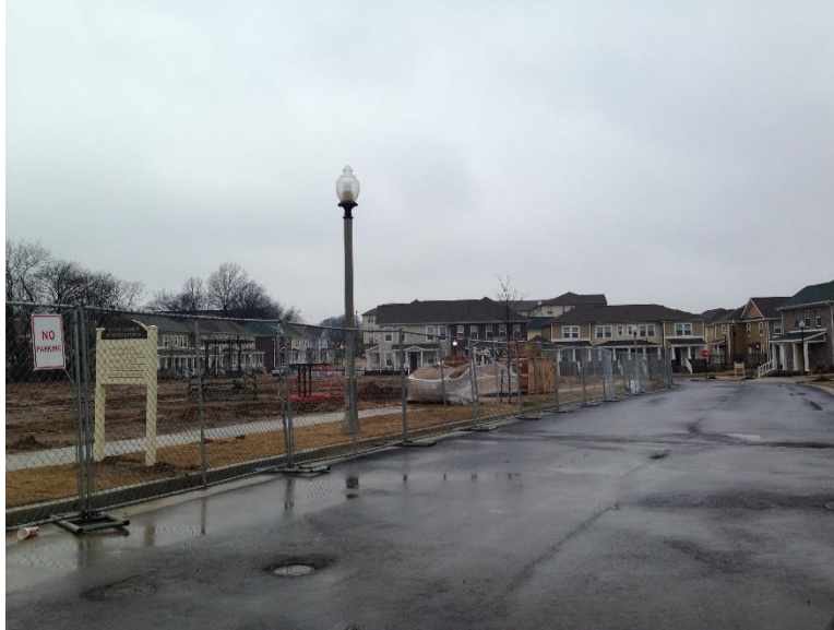
A.23 Ongoing Construction at Cleaborn Point (C. Wommack 2015)
