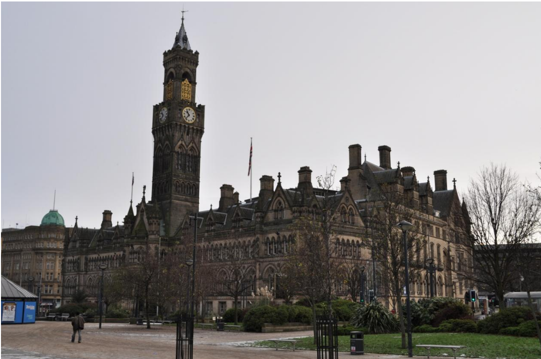
Picture 3-6: Bradford City Hall in Centenary Square where surveys were conducted (Reid, 2010)
