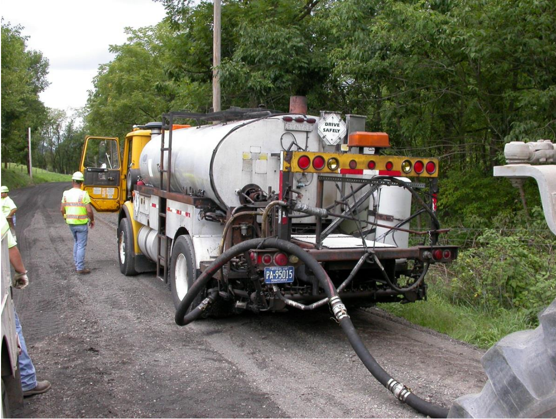
Figure 2:6: Emulsion truck connected to the reclaimer (Morian et al. 2012)
