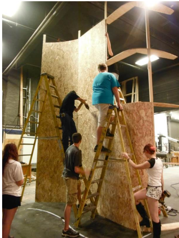
Figure 32. Covering the “ribs” with Oriented Strand Board. Photo taken by Ashley De Lys Harman: September 2012
