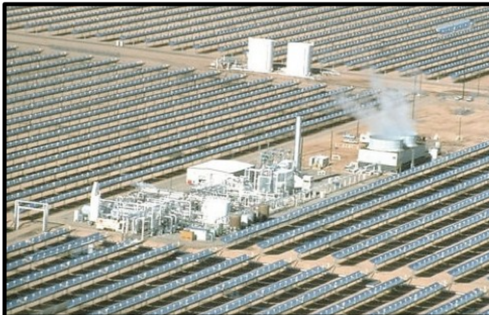
Figure 16: 10 MW SEGS I Power Plant and Trough Array in California (NREL, Parabolic Trough Power Plant System Technology, 2010)
