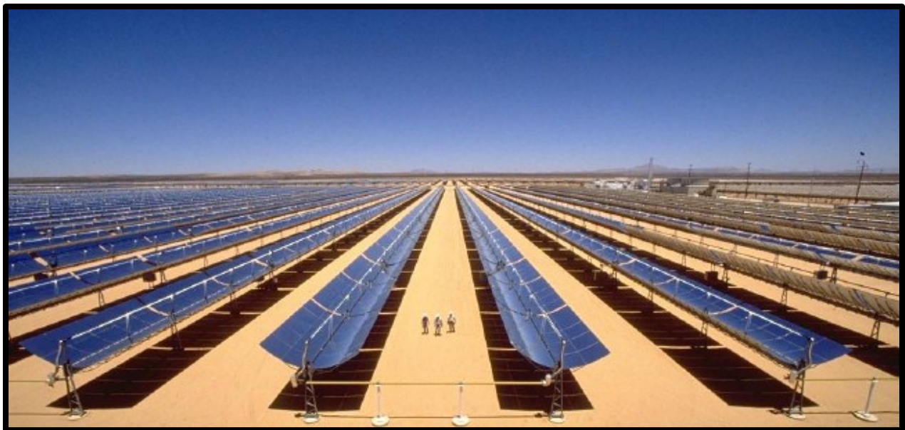
Figure 3: Parabolic Troughs from the 280 MW Power Plant Solana under Construction in Gila Bend, AZ (Siemens, 2009).
