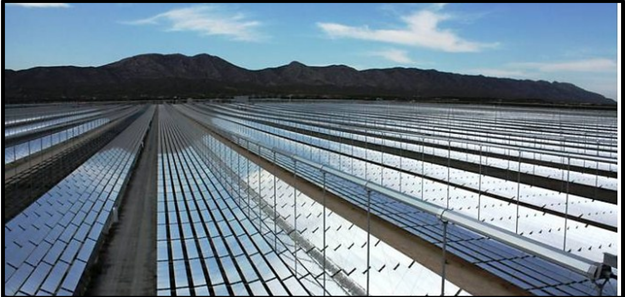
Figure 4: Linear Fresnel Array at the 30 MW Puerto Errado 2 CSP Plant in Calasparra, Spain (PE2, 2010)
