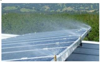
*Figure 6: Heliotex sprinkler system*<sup>8</sup>(*Reproduced without permission*)
