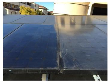
Figure 42: Cleaned panel (left) vs. Soiled panel (right)
