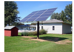
Array Tech Inc., DuraTrack DA Solar Tracker
