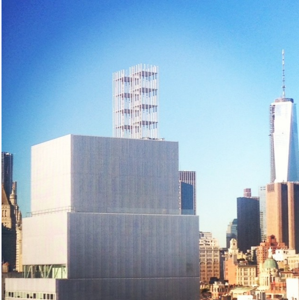
Figure 17: Chris Burden, Two Quasi-Legal Skyscrapers , 2013. New Museum, New York. Structural aluminum framing, glass, wood 2 x 4s, steel hardware (stainless steel cable, turnbuckles, clis and angles, t-nuts, half-inch bolts) Image source: http://www.newmuseum.org/blog/view/chris-burden-at-the-juncture-of-art-and-architecture-collaboration-and-risk (accessed April 11, 2017)
