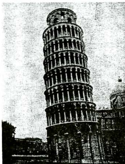
Fig. 1. The Leaning Tower of Pisa
