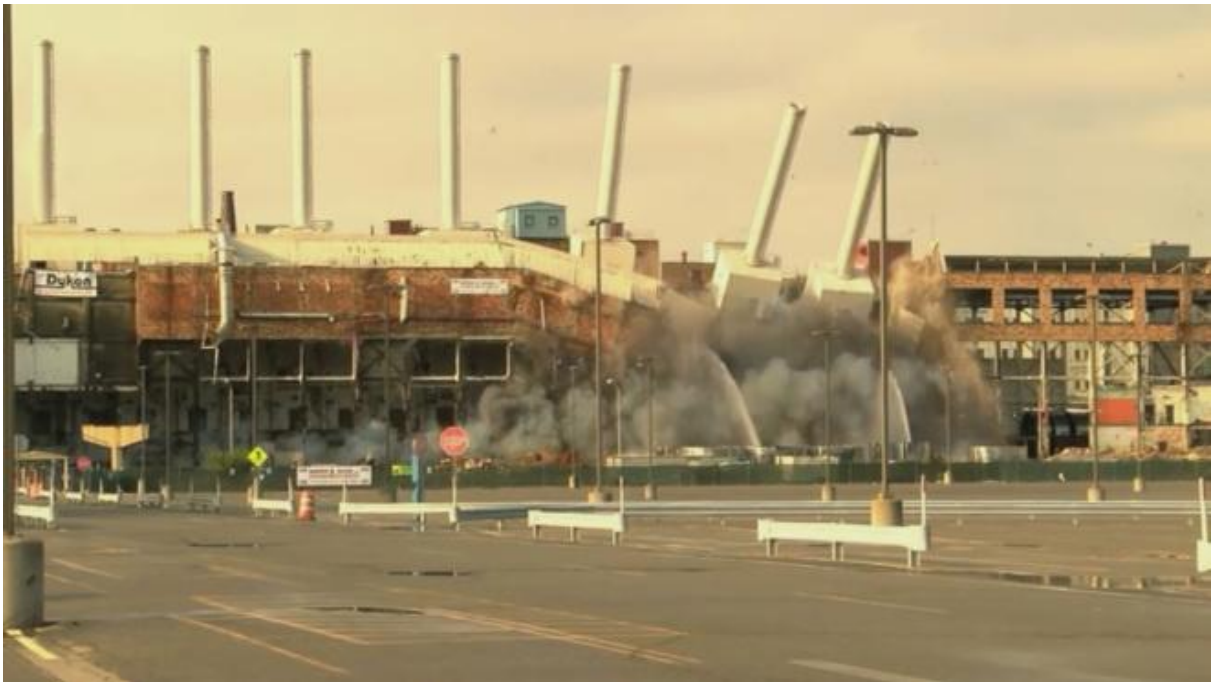
Fig. 2. Demolishing 92-year-old Kodak Building in Rochester, New York, 2015
