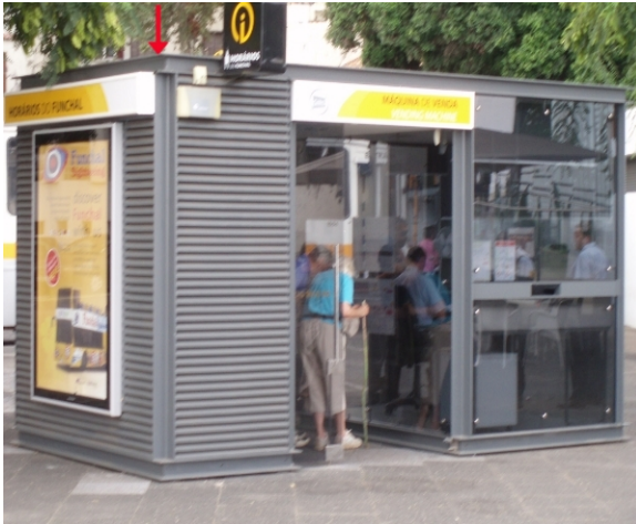
(a) Installation location
