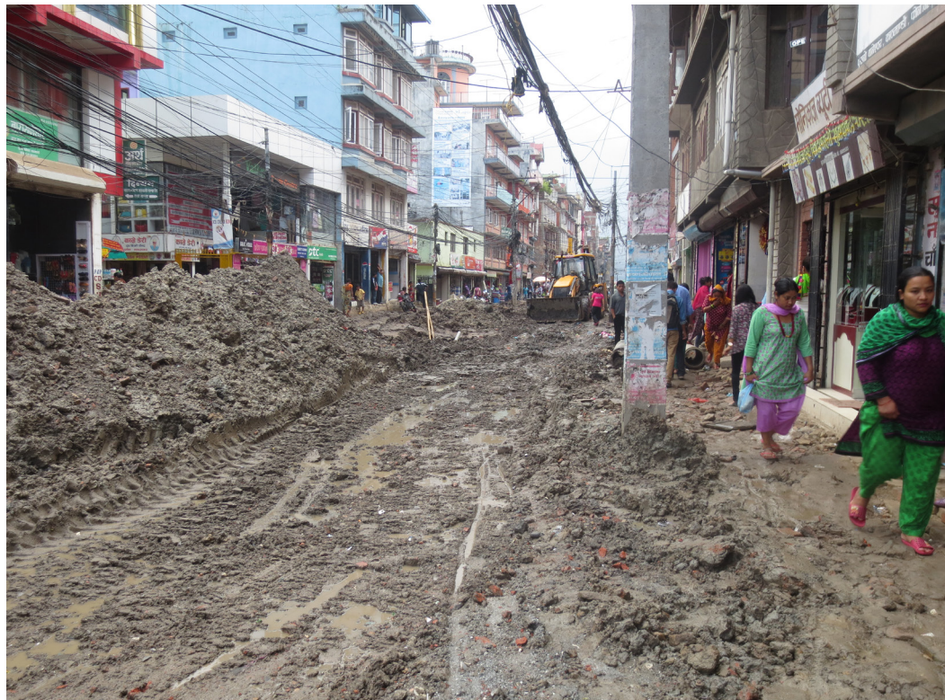
Figure 1. Road from Purano Baneshwor to Sinamangal.
