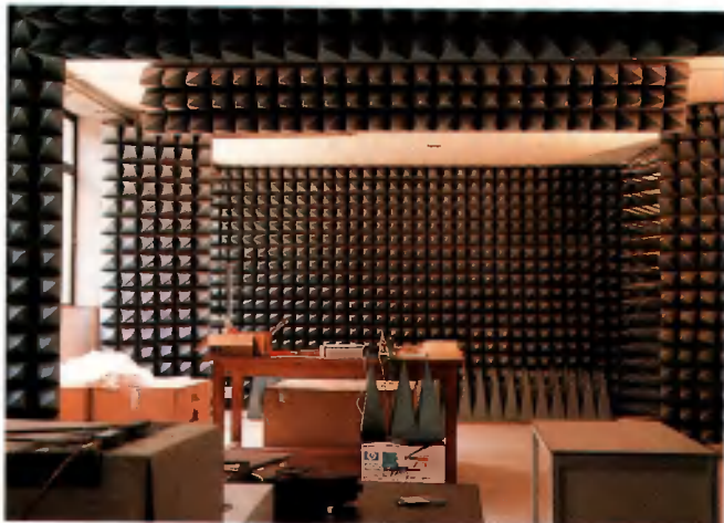
Fig. 61: Works in progress for the implementation of the Interim Laboratory.
