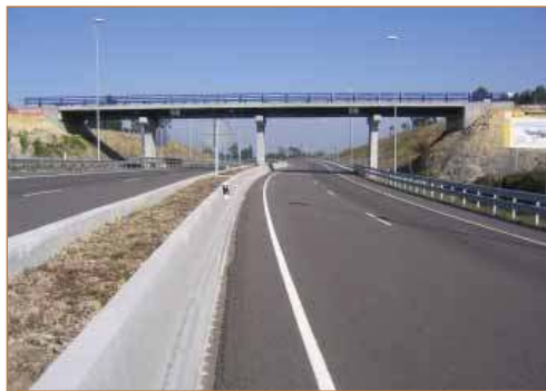
The first European fully vehicular highway carbon fibre composite bridge was installed in Spain
