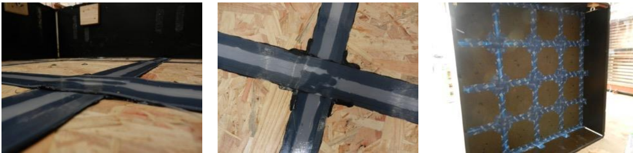
Fig. 7: Impact of crossings; left: openings at crossings silicone strip; middle: addition of silicone at crossings; right: addition of crosses of tape at crossings
